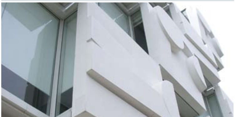
Cultural patterning references in facade design create a distinctive city centre.
